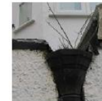
Blocked hopper head
